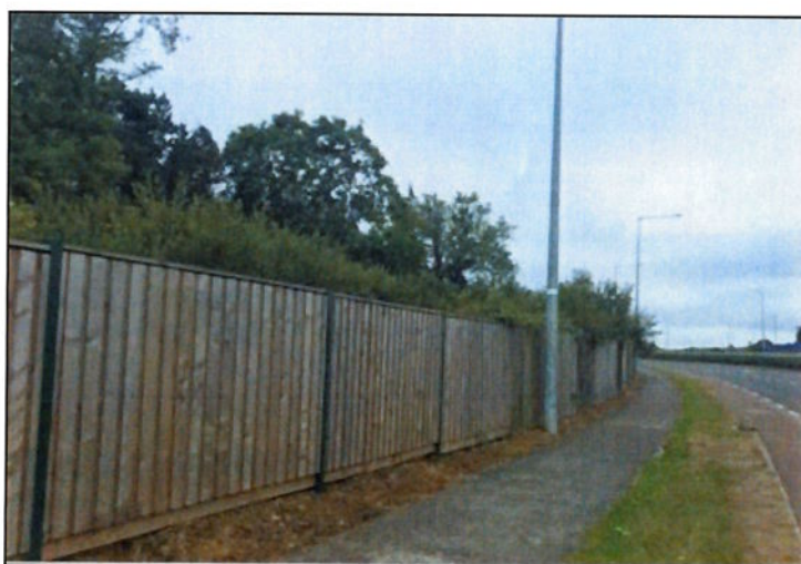
Plate 4.3: Fencing along western perimeter
